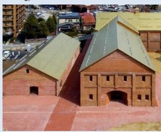
PFI Project for Development of Surrounding Area of Yoshino-cho Ryokuchi in Hirosaki City Hirosaki-shi, Aomori Public facility (art museum) Facilities by private sectors (museum shop, café, cider mill) Grand opening in July 2020
