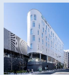
Yokohama Cultural Gymnasium Redevelopment Project For profit private sector facility (hotel, etc.) Yokohama-shi, Kanagawa Hotels, restaurants and large bath Opened in April 2024
