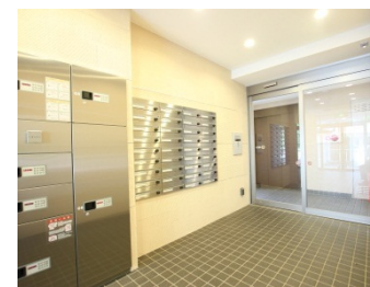
Installation of parcel delivery boxes
