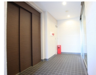
Installation of automatic lock system
