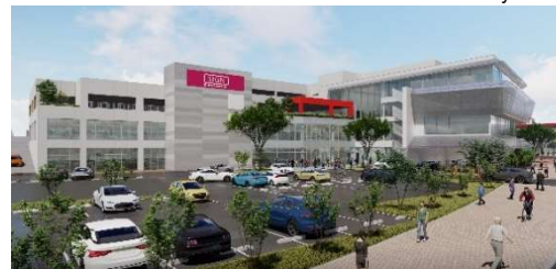
Urban planning road on the north side
