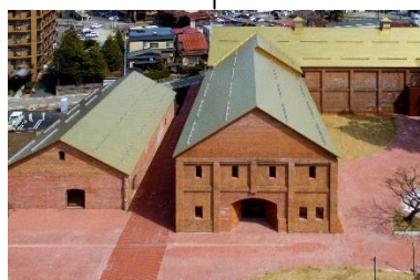
PFI Project for Development of Surrounding area of Yoshino-cho Ryokuchi in Hirosaki City Hirosaki City, Aomori Prefecture Public facility (art museum) Facilities by private sectors (museum shop, café, cider mill) Grand opening in July 2020
