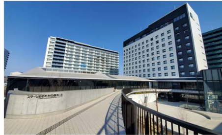
City-Owned Land Development Project in Front of Nagareyama-Otakanomori Station Nagareyama City, Chiba Prefecture Public facility, hotel, apartment Opened in January 2019 (hotel building) Opened in April 2019 (public facility building) Completed and handed off in March 2020 (apartment building)
